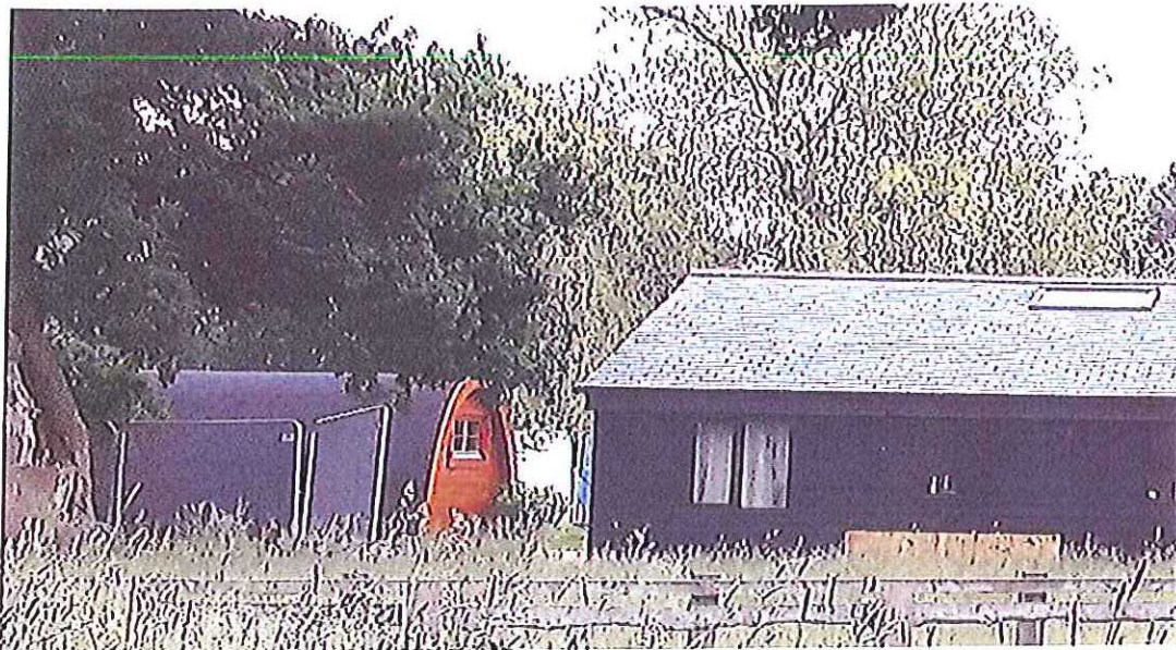
Picture showing breach of security fence, and evidence of security fencing not being provided as a condition of the licence between the event and properties to the west
